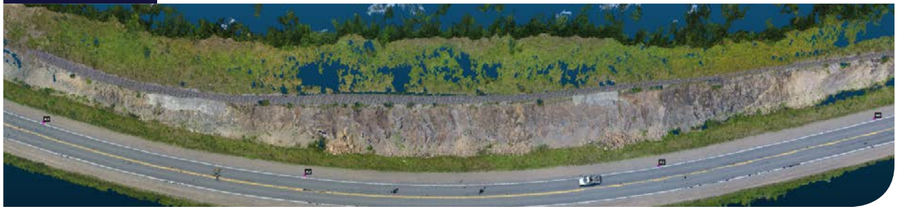
Figure 16 UAV point cloud of entire wall
