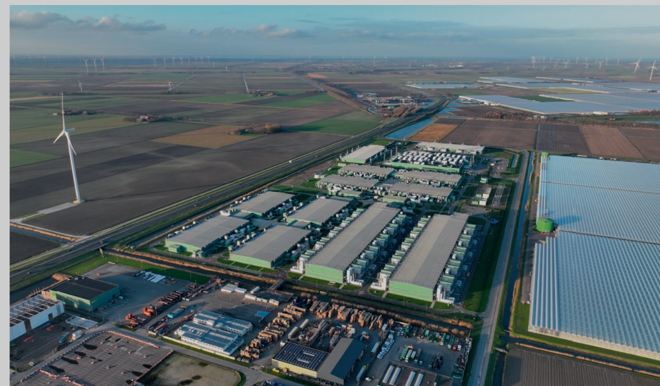
Aerial view of Microsoft data centre in Middenmeer, the Netherlands
