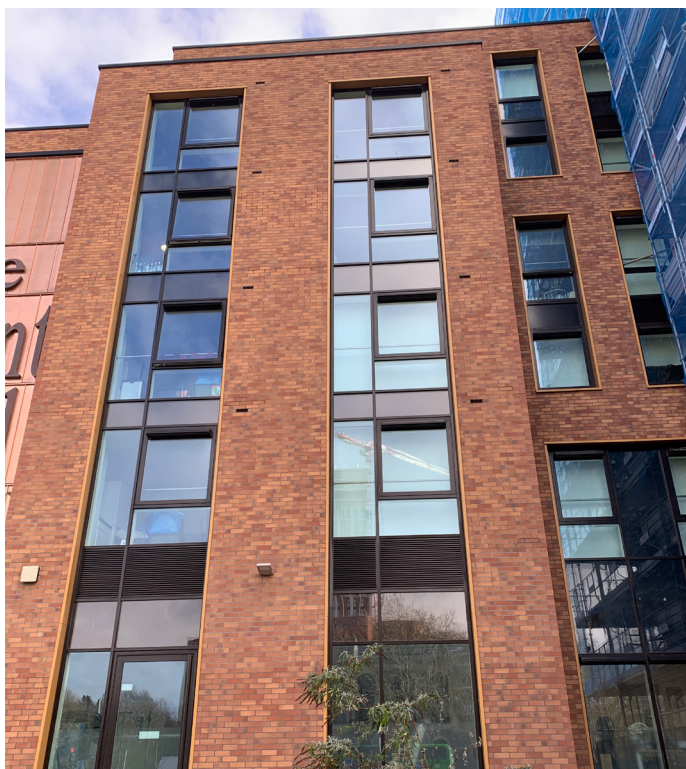
Figure 21: Brick slip façade
