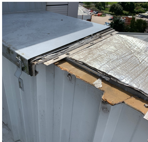
Figure 14: Typical metal insulated panels with PIR/PUR core
