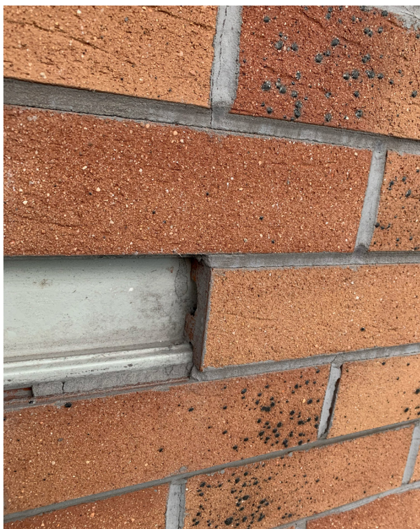
Figure 20: Close-up view of brick slip system
