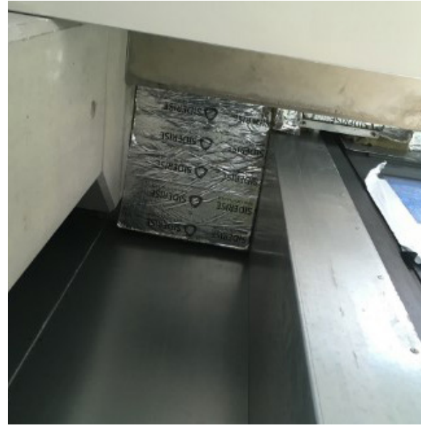
Figure 2: Typical horizontal fire-stops with smoke foil
