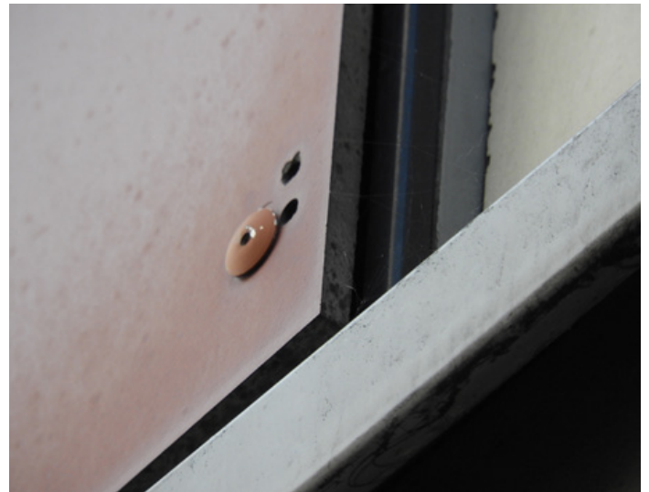
Figure 18: Close-up view of HPL cladding panel
